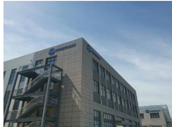
Plant Extension in Changzhou, China
