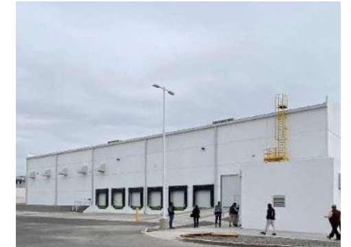
Warehouse, Dock & Label Printing Room
