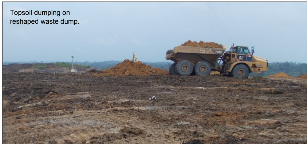
Figure 5.3 – Topsoil Handling and Rehabilitation
