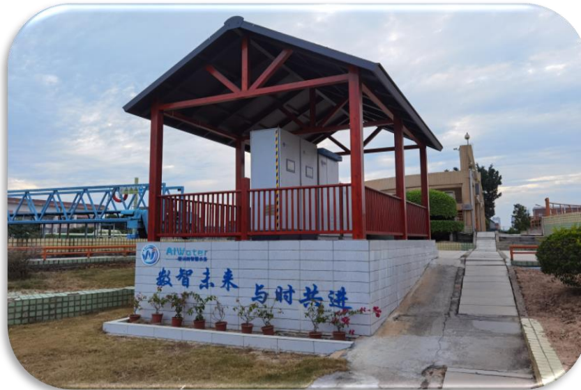
Installation of AIWater Control and Instrumentation Systems at Plant A.
