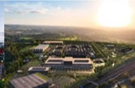
AiOnX data centre development fund
