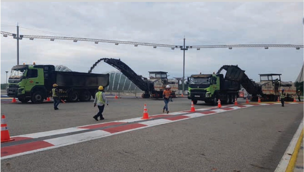
Supply and Lay of Asphalt Premix
