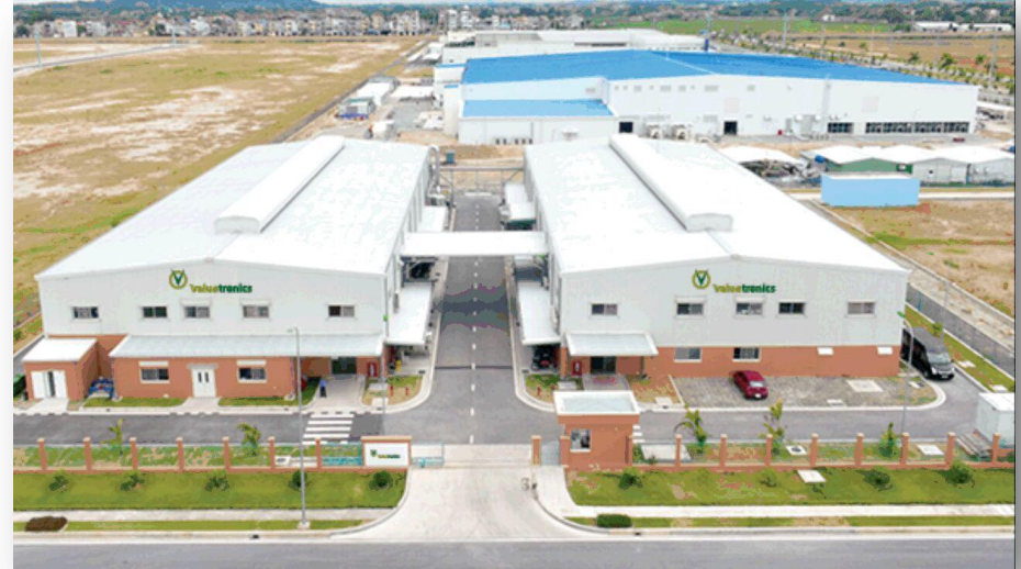
Phase II - Leased standard factory (Trial production started in May 2020)
