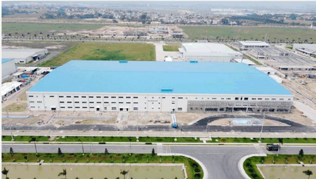
Phase III - Vietnam Campus (Expected to commence production by the end of FY2022) Located in the same reputable Japanese run Industrial Park as Phase II. Land area: 52,541 sqm.
