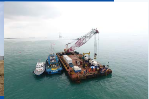
Marine Civil Works – Cable/Pipe Laying
