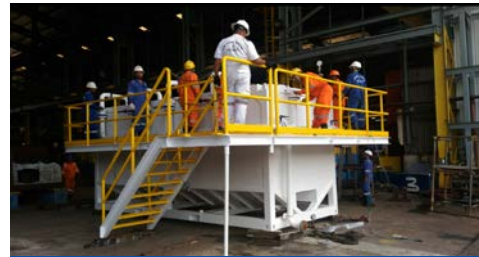
Fabrication of Dehydrator Tank
