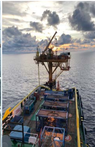
Offshore Platform Maintenance Work
