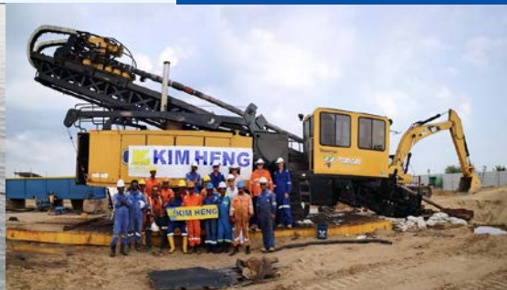
Horizontal Directional Drilling (HDD)
