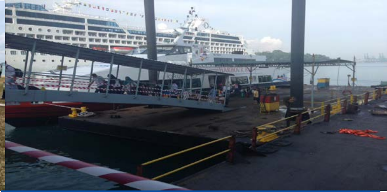
Fabrication & Supply of Landing Spud Barges to Cruise Terminal
