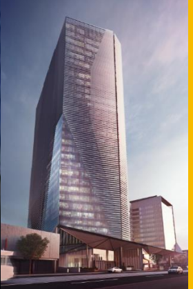
311 Spencer Street, Melbourne (50% interest) -Under construction-
