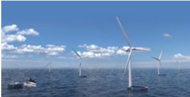
Seatrium's Small Waterplane Area Cylindrical Hull (SWACH) is one of the novel solutions for floating offshore wind turbine foundations. We partnered with TCOMS to validate computational models through scaled-down model tests.
