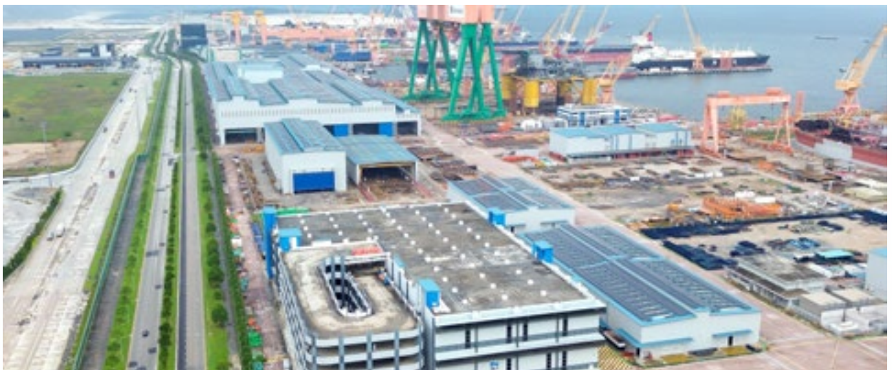
In 2023, we have expanded the capacity of the solar panels installed at our Tuas Boulevard Yard from 8.5MWp to 10.5MWp
