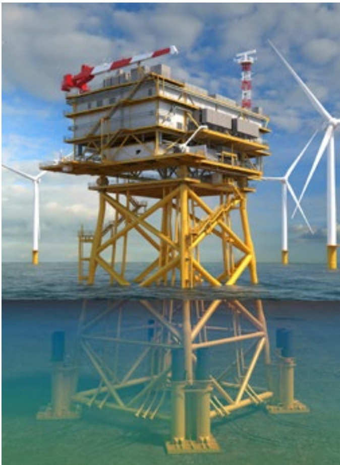
Awarded a contract for the engineering, procurement and construction of an offshore substation for Empire Wind 1 in May 2023: This project further demonstrates our capabilities in the renewable energy sector, as we contribute to the development of offshore wind infrastructure for Empire Wind 1
