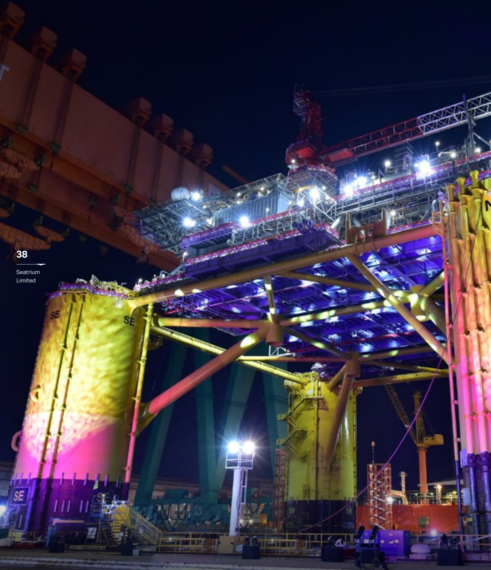
Whale FPU, second FPU delivered on time and within budget to Shell Offshore, for deployment in the Gulf of Mexico
