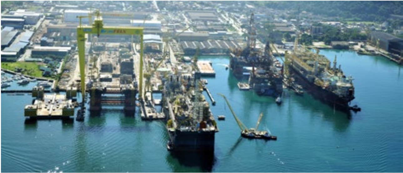
Our Aracruz Yard and Angra Yard (top), tapped on renewable electricity sources, increasing the share of renewable energy in our energy mix
