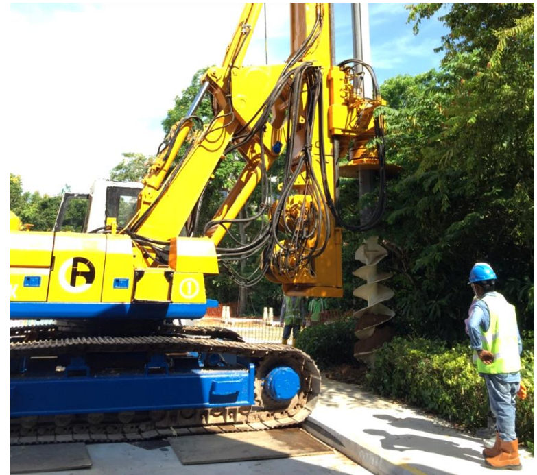
Driving the first pile into the ground
