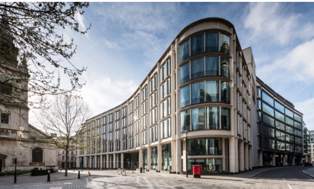
Full occupancy achieved in 30 Gresham Street, London
