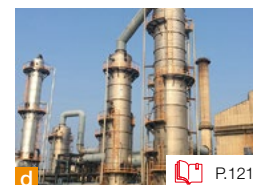
d Facility that uses CO 2 capture technologies supplied by Carbon Clean Ltd.
