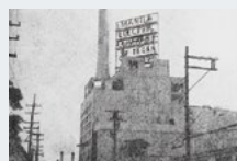
Manila Electric Company's generator No. 1 (Philippines)
