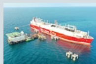
Jawa-1 Gas-to-Power Project (Gas-fired power plant and floating storage and regasification unit (FSRU)) (Indonesia)
