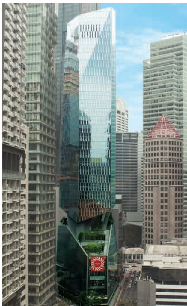
The brilliance of 18 Robinson is accentuated by its shimmering glass facade
