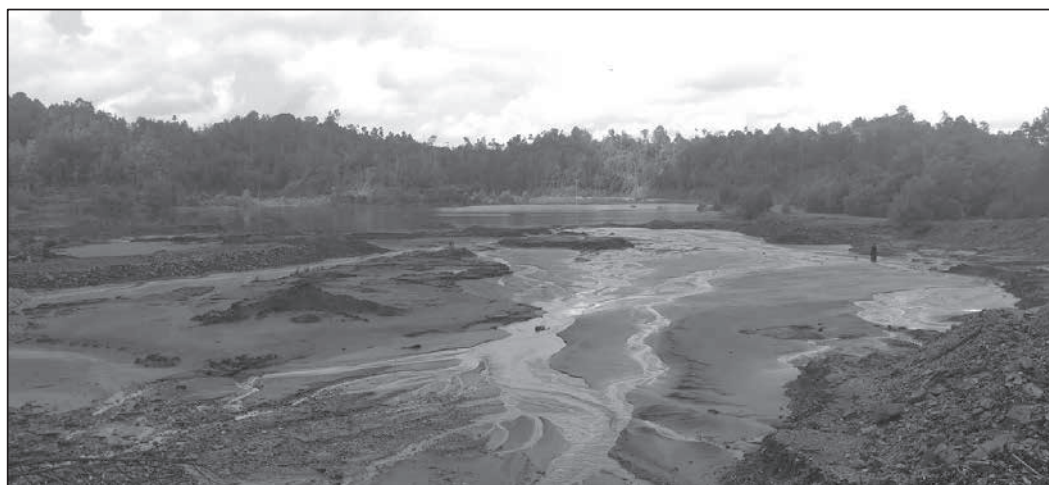
Figure 10.2 Lubak Mandi tailings dam looking southwest
