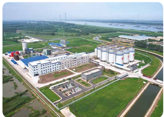
Integrated manufacturing complex in Jingzhou, China.
