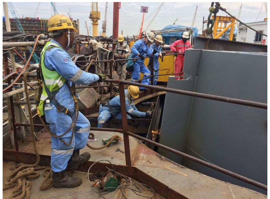
Above: Safety harnesses is a must for workers when working in height on-board vessels. Below: A worker welding, with a team of supervisor and safety officers doing their safety inspection rounds. All of them had donned their safety equipment.
