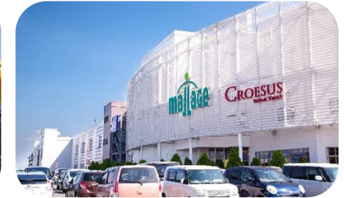
Mallage Shobu Suburban shopping centre in Kuki city, Saitama Pref.
