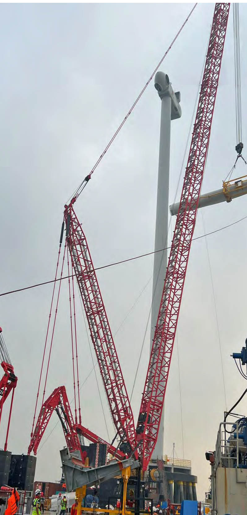
Installation of wind turbine using our 1250-ton crane in Vietnam
