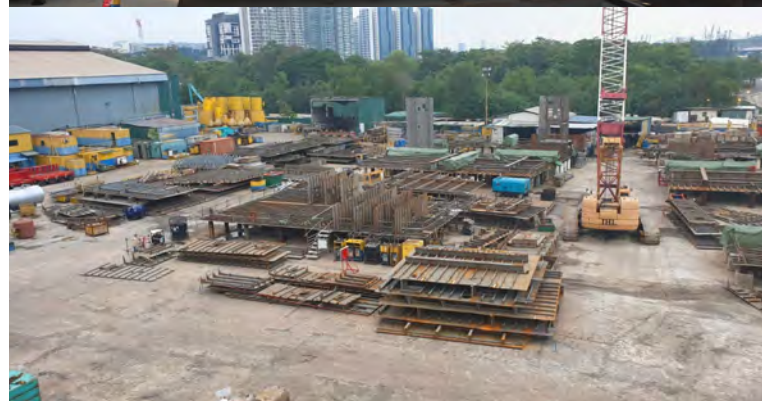
Hull block fabrication at Kim Heng yard
