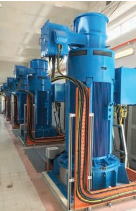
Pumpsets replacement at Choa Chu Kang Waterworks .
