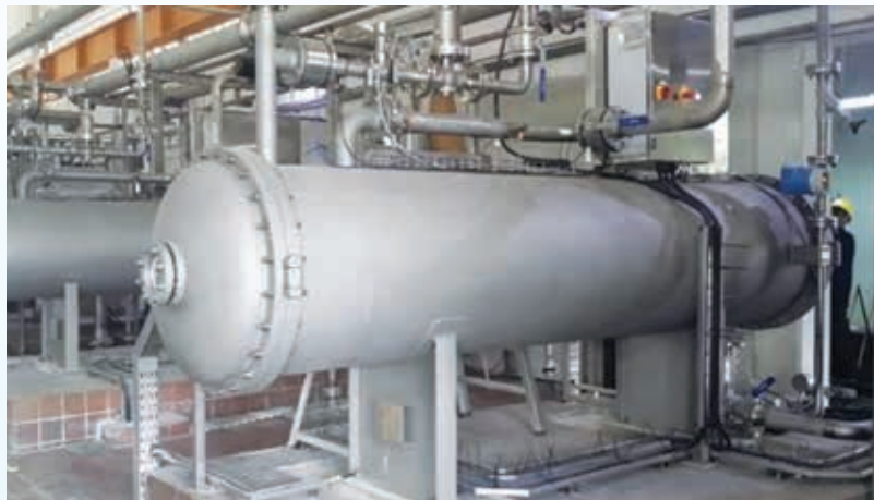
Ozone Generator System Replacement at Bedok Waterworks .
