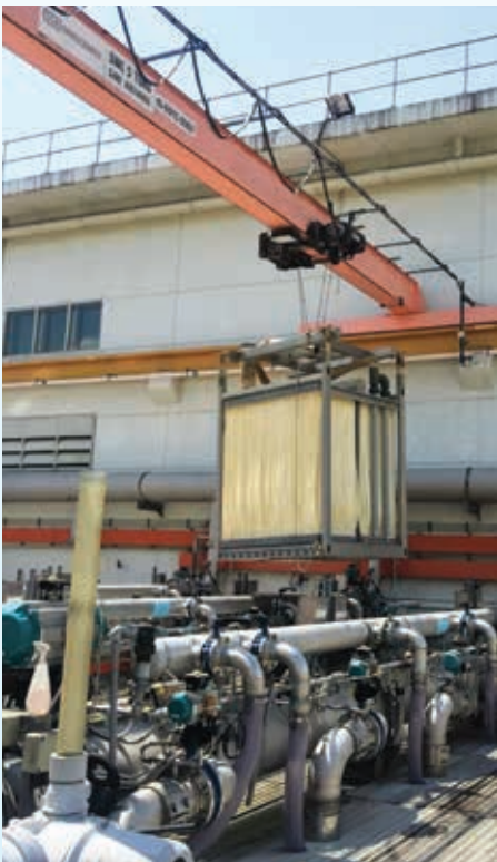
Ultrafiltration Membrane Replacement at Chestnut Avenue Waterworks .
