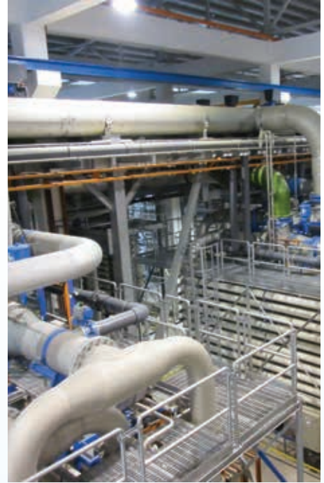
Civil, Mechanical and Electrical Works at Lower Seletar Waterworks .
