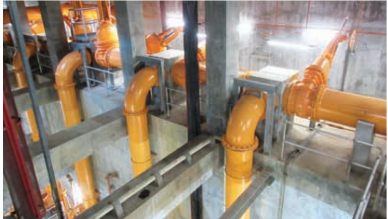
Renewal of Equipment and Upgrading of Water Pumping Installations at Choa Chu Kang Pumping Station .
