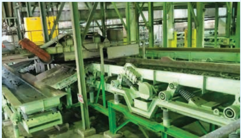
Vibration Conveyor System Replacement at Tuas South Incineration Plant .
