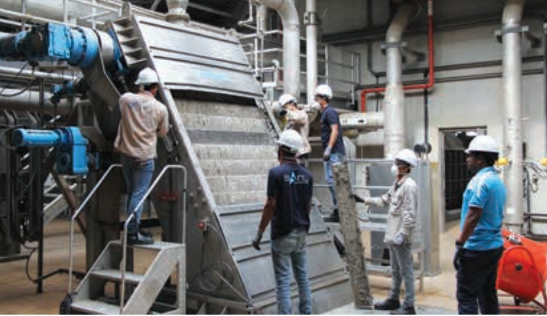
Servicing and Maintenance of Screening Sludge, Grit and Related Equipment at Changi Water Reclamation Plant .
