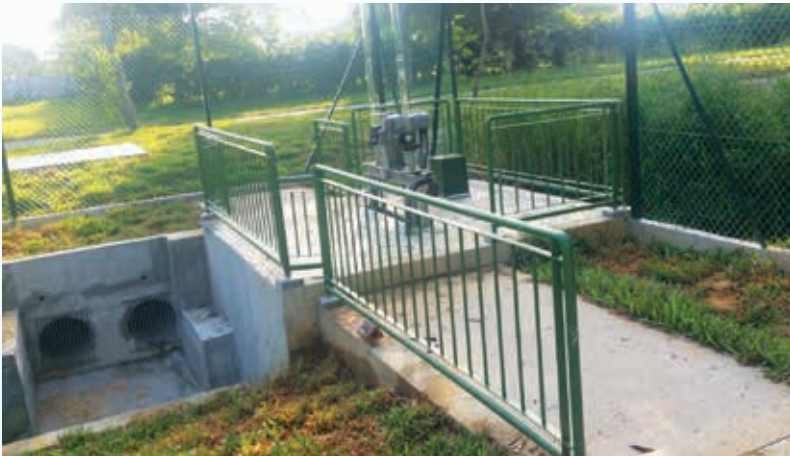
Construction of Drains and Supply of Pumps at Lorong Halus .
