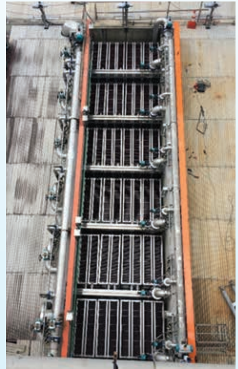
Construction of Ceramic Ultrafiltration Membrane System at Chestnut Avenue Waterworks .
