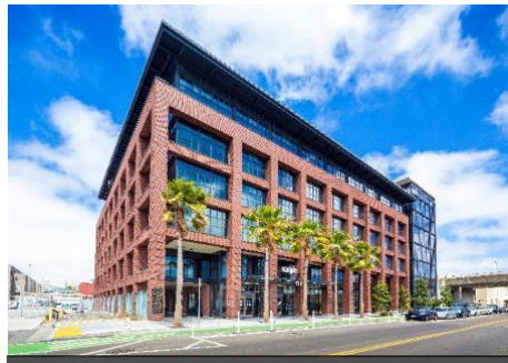
510 Townsend Street, San Francisco, US
