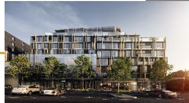
Adina Apartment Hotel Melbourne West End
