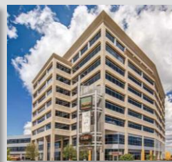
VILLAGE CENTER STATION I Denver, Colorado
