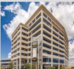
VILLAGE CENTER STATION I Denver, Colorado
