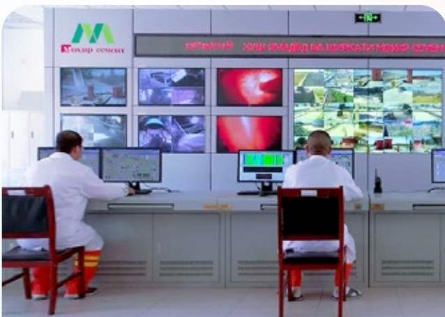
Central Control Room of IMCCMC
