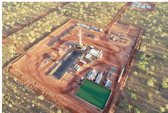
Kyalla 117 well site
