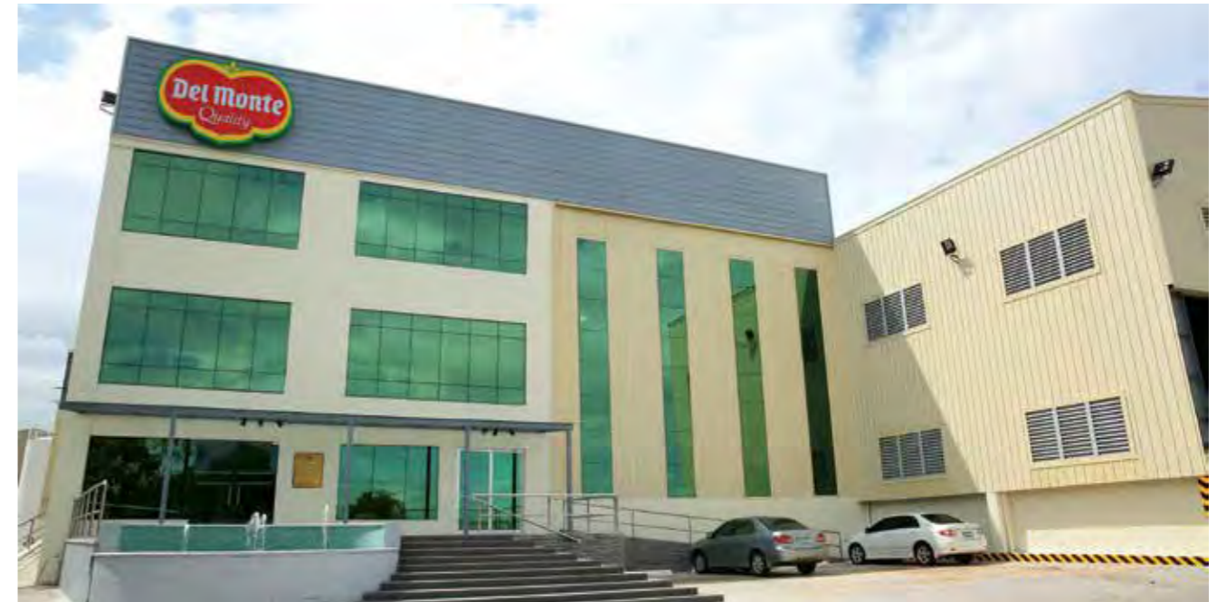
Del Monte Philippines Beverage plant in Laguna, Philippines
