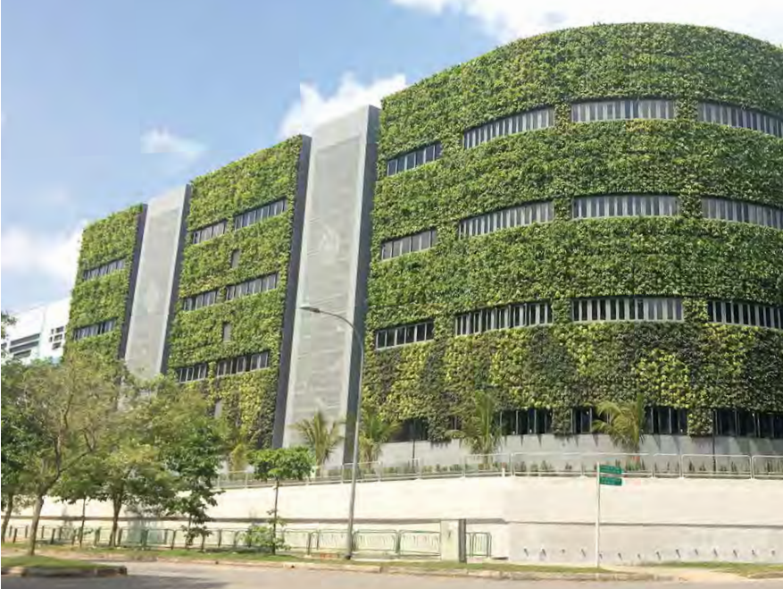
HKF Office Warehouse
