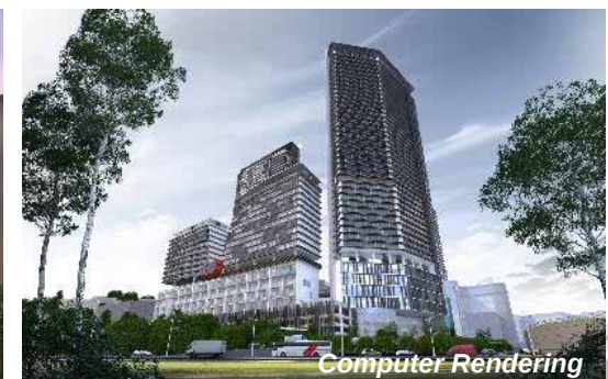
Mixed-use development in Selangor
