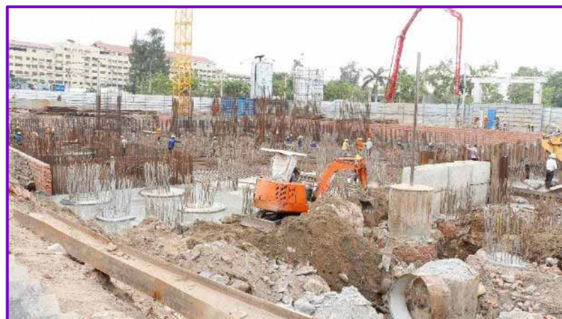
Construction Update as of April'15
