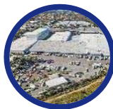
69 Sargents Road, Minchinbury
