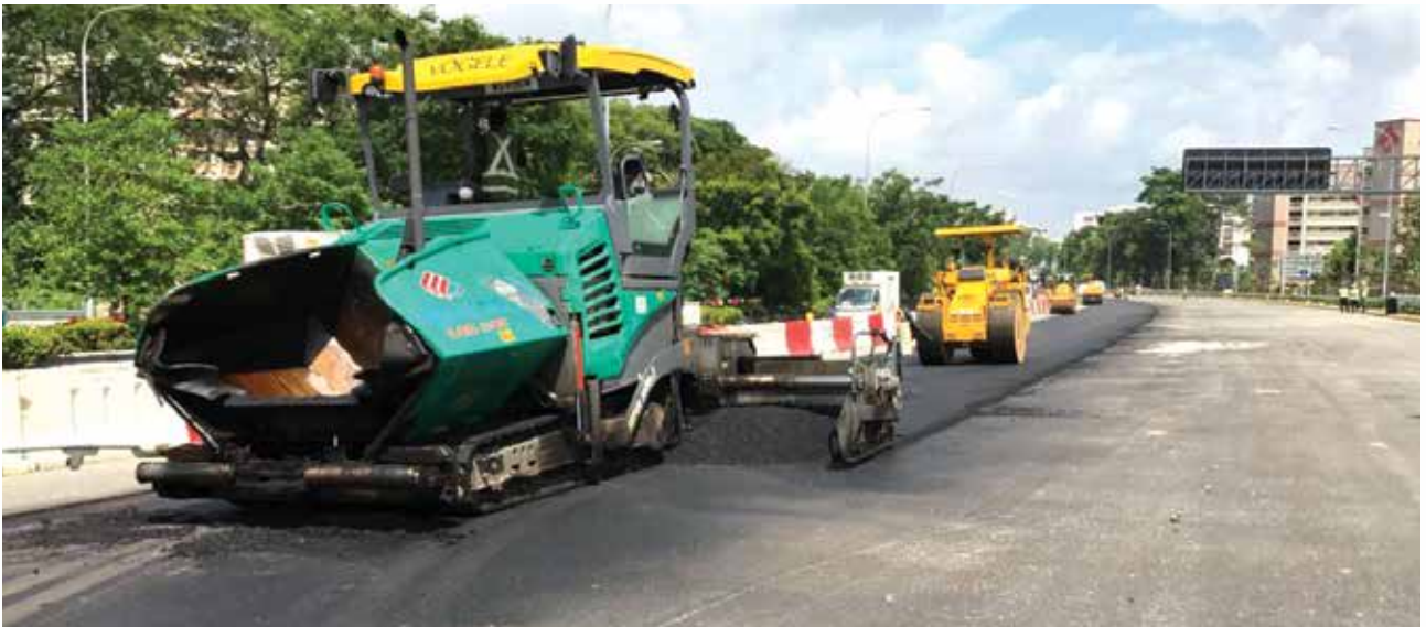
▲ Supply and lay of asphalt premix
