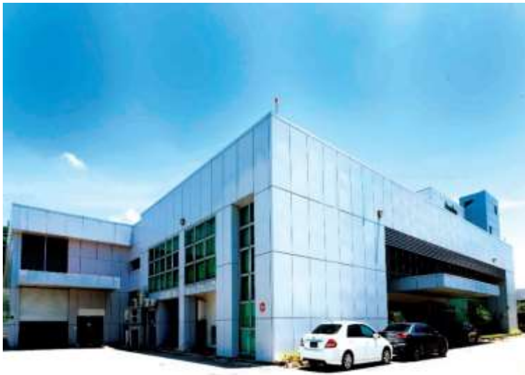
19 Changi South Street 1
