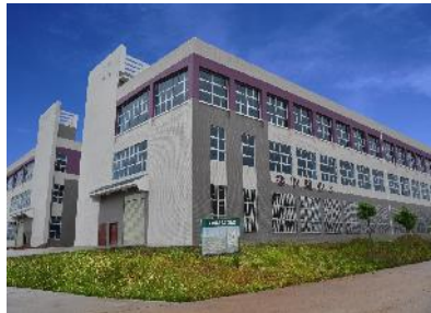
Completed factory of Fujian Zilaohu in Liancheng Industrial Park, Food Processing Area will be operational by end of March 2017.
