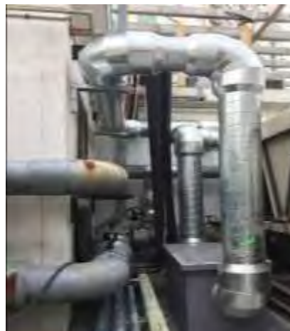
INSTALLATION OF NEW CHILLED WATER PIPES FROM TROPICANA CITY MALL'S CENTRAL CHILLER PLANT ROOM TO TROPICANA CITY OFFICE TOWER
