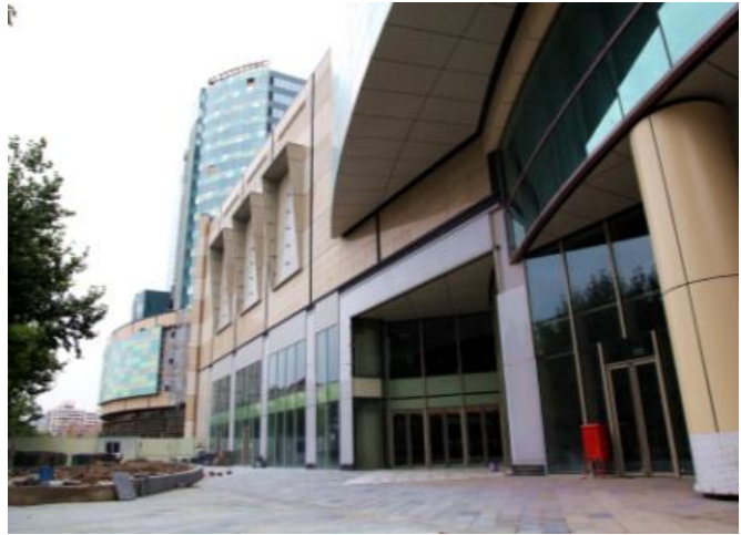
External landscape work of TP1 completed
