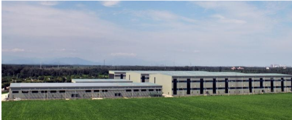
Aerial View of Beijing Logistics Park
