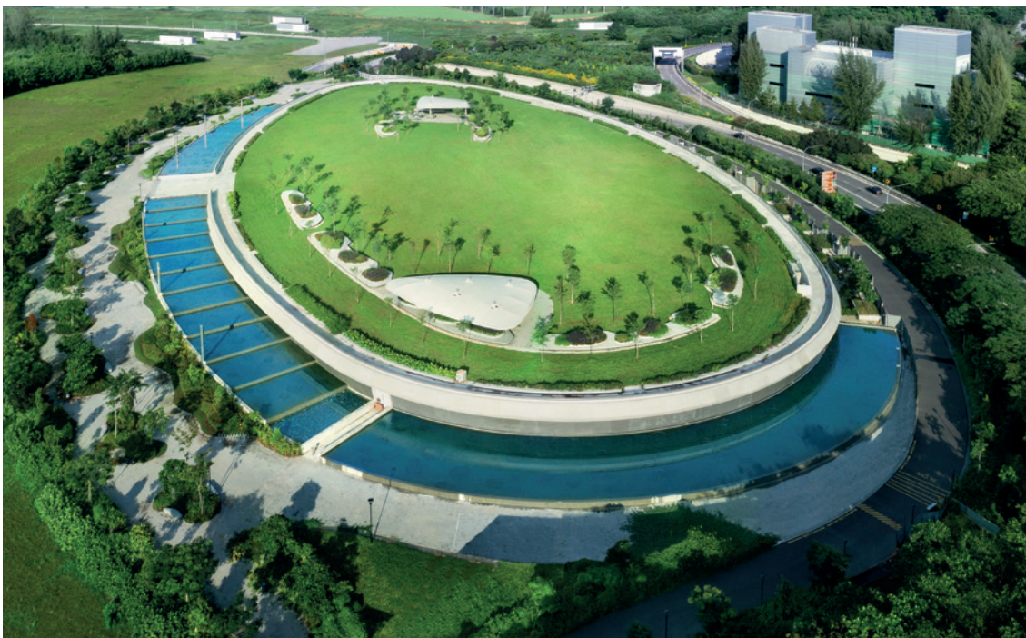
Keppel Marina East Desalination Plant, Singapore's first large-scale, dual-mode desalination plant, which is developed and operated by Keppel.
