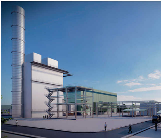
The global transition away from fossil fuels and towards zero- and low-emission technologies bodes well for many of the solutions that Keppel provides, including renewables and the development of the Keppel Sakra Cogen Plant, Singapore’s first hydrogen-ready and most advanced power plant (in picture).
