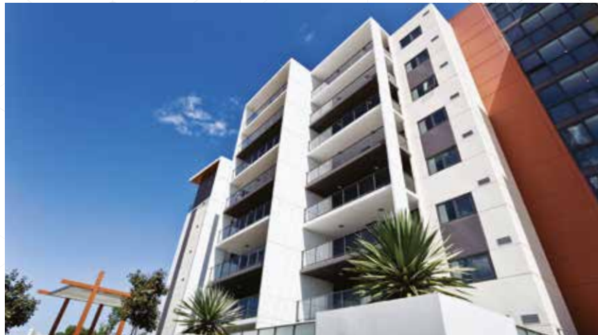
Looking up at Unison on Tenth tower from landscape deck
