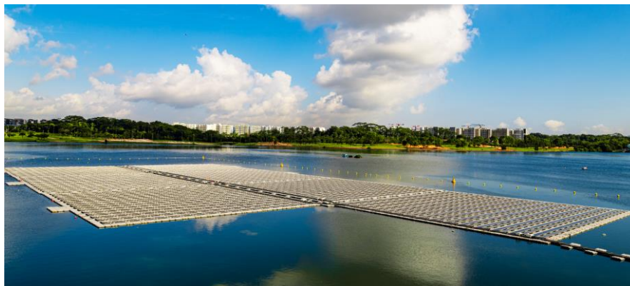
Floating Solar PV Systems at Bedok Reservoir (top) and Lower Seletar Reservoir (bottom)
