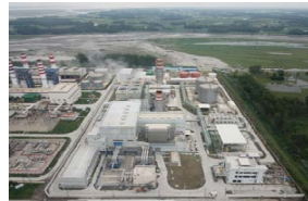
The Sirajganj Unit 4 combined cycle gas turbine power plant in Bangladesh commenced commercial operations in 2019
