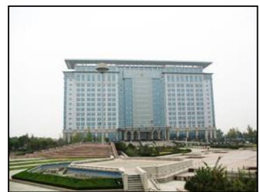
Jiaozhou Municipal Government Building of Shandong Province (山东省胶州市政府大楼)
