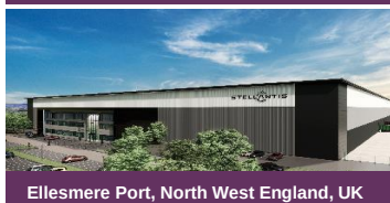
Ellesmere Port, North West England, UK
