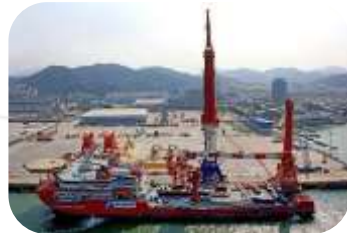
Installation of Huisman crane
