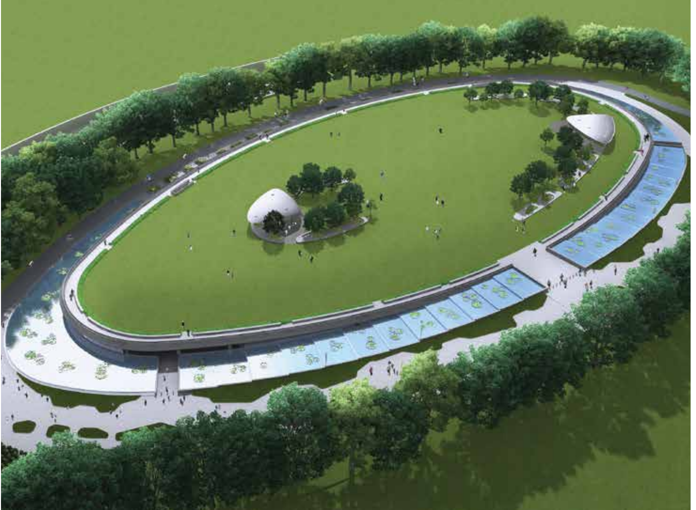
Marina East Desalination Plant photo courtesy of Keppel
