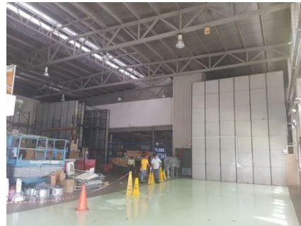
1st Storey - Warehouse area
