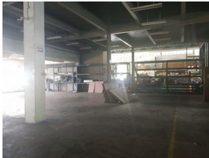
1st Storey - Warehouse area
