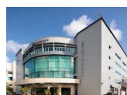
25 Changi South Ave 2
