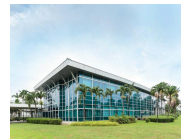
3 Tuas South Ave 4
