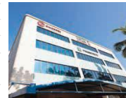
31 Changi South Ave 2
