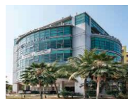
2 Tuas South Ave 2
