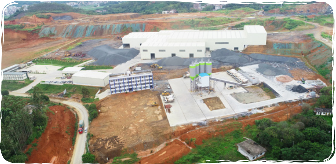
Construction waste material recycling facility and Cenxi Xing Jian ready-mix concrete manufacturing facility
