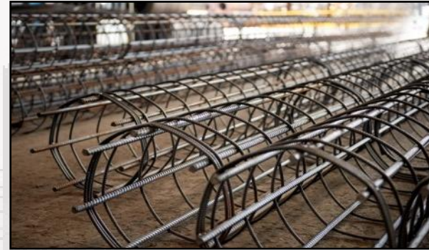
Pre-fabricated Cage (Bored Pile Cage)
