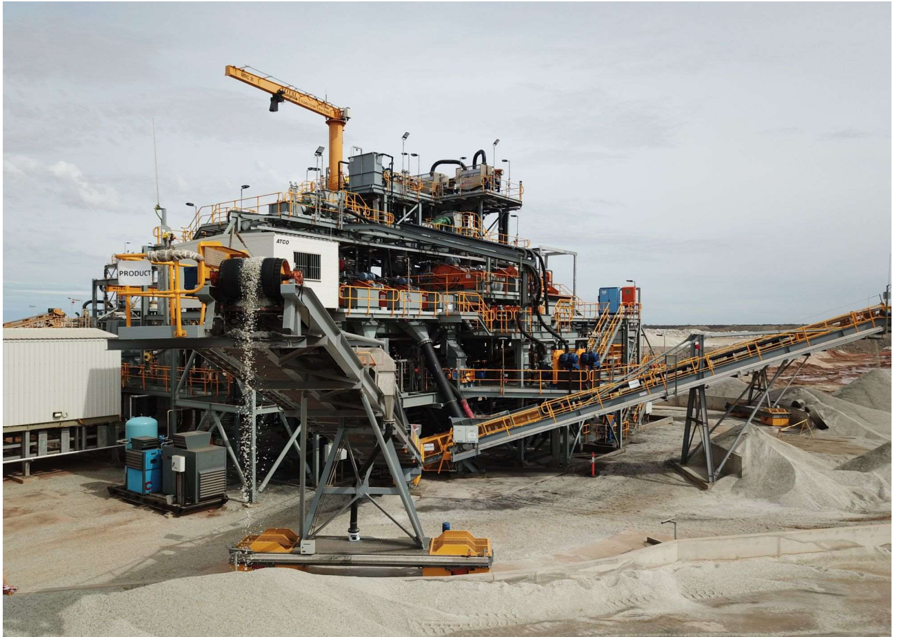
Figure 3: Stage 1 DMS Plant
