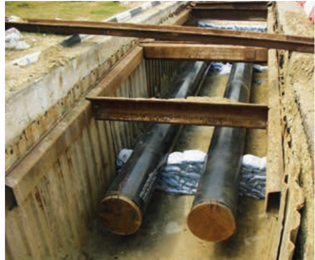
Worksite – laying of gas pipe
