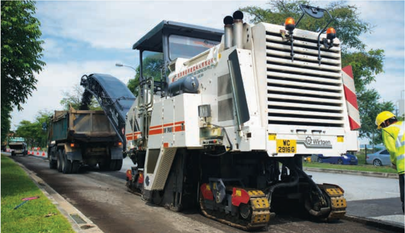
Worksite – road maintenance
