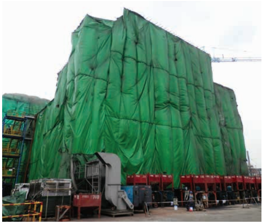
Modules covered with canvas during blasting process
