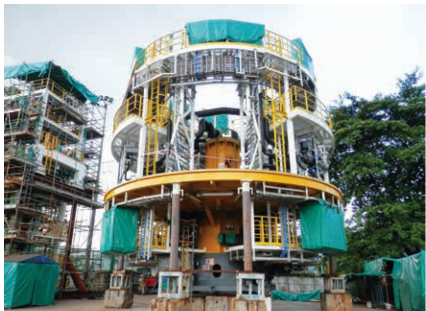
Assembly of GEO Stationery Turret in progress
