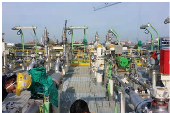
Top deck of a topside module
