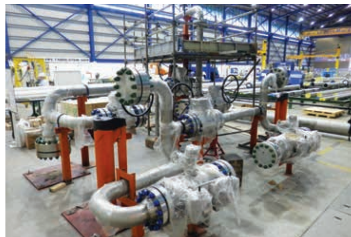
Piping works in our workshop
