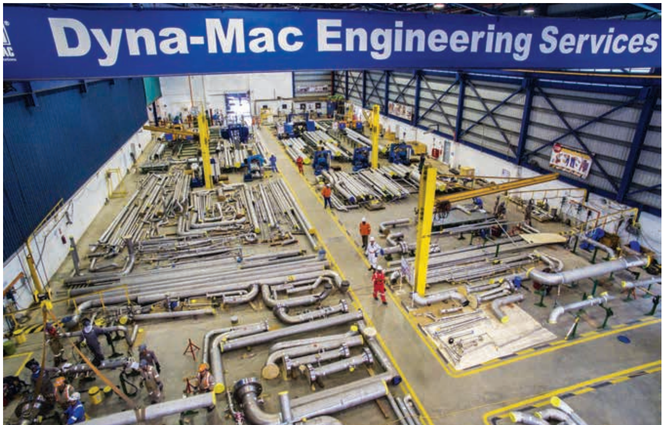
Our piping workshop at West-Yard
