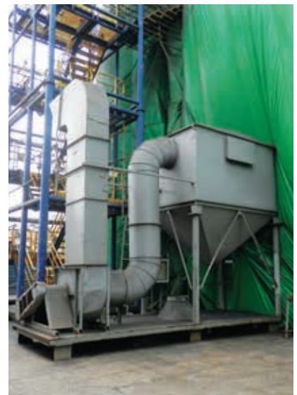
Dust collectors during blasting process
