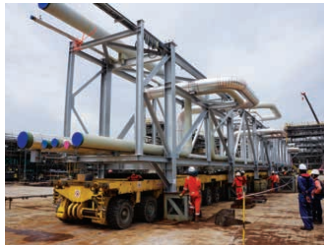
Pipe tracks being transported to sea-front for load-out
