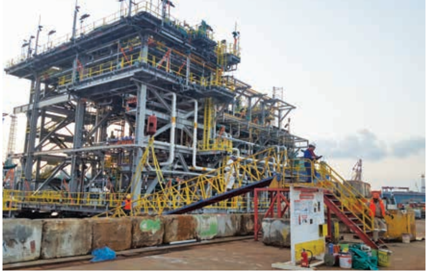
Load-out of Topside module
