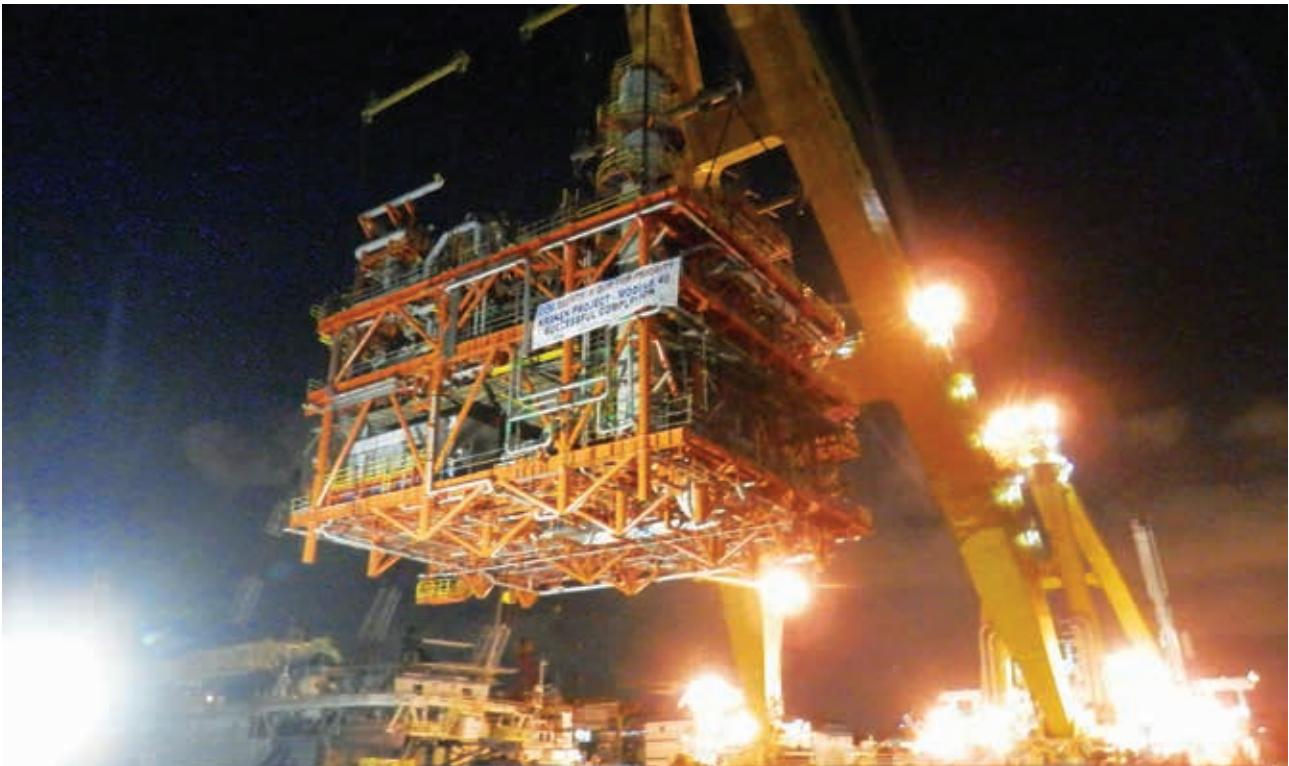
Load-out of topside module
