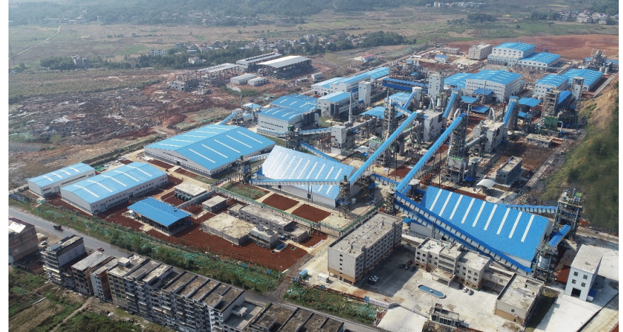
JBJLIL Conversion Facility
